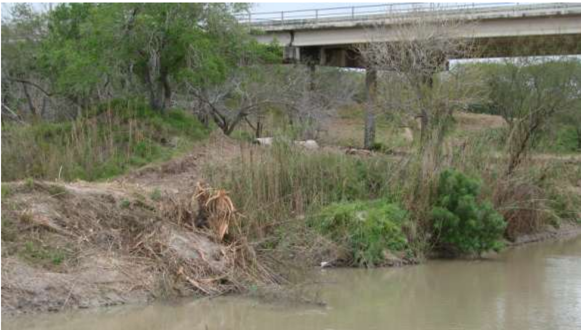
Damage on an Arroyo bank.
