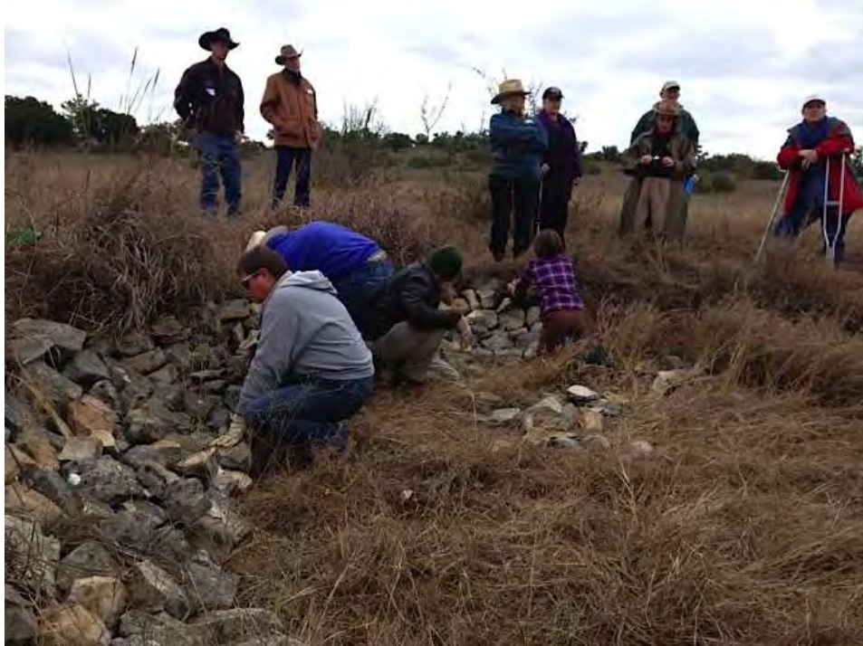
Participants laying stones to slow field erosion by stopping a head cut on the Williams property at the Land Health Workshop while other participants and Quivira Coalition coordinator, Mollie Walton, look on.
